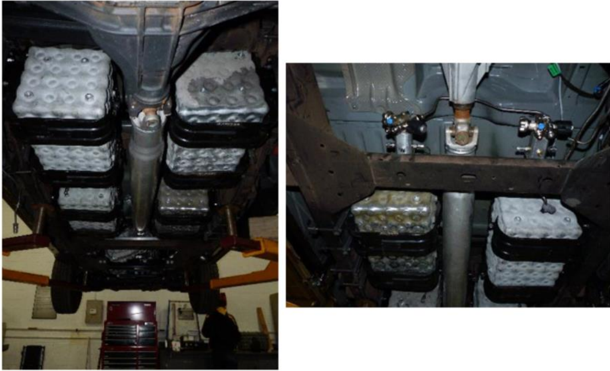
Figure 17- Tanks installed in the truck chassis [6]
